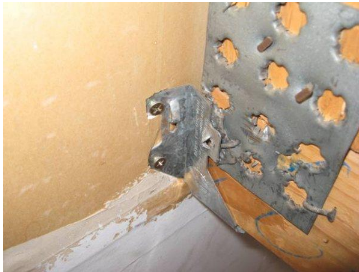
Above: gang-nail integrity destroyed
