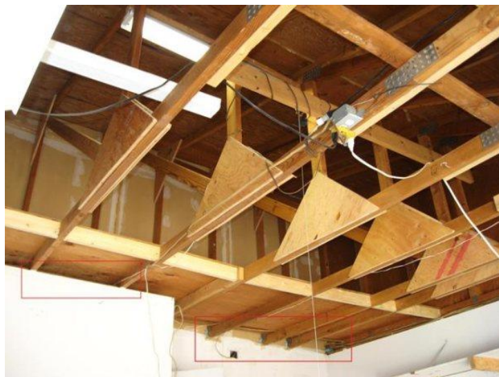
Above: trusses and truss connections
